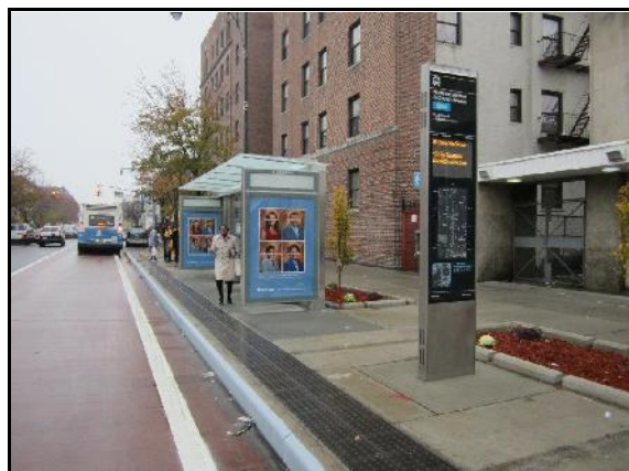
Completed Select Bus Service Station on Nostrand Avenue between Church Avenue and Erasmus Street
