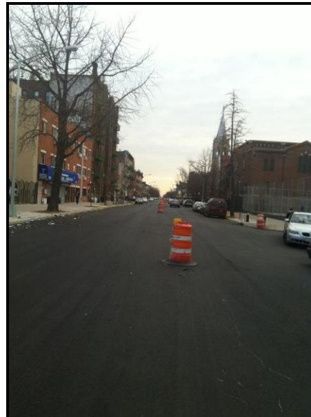
Paved Roadway - Church Avenue between Rogers Avenue and Bedford Avenue.
