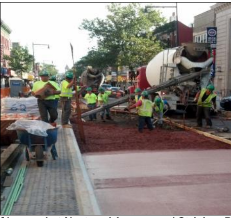
Installation of bus pad at Nostrand Avenue and St Johns Place
