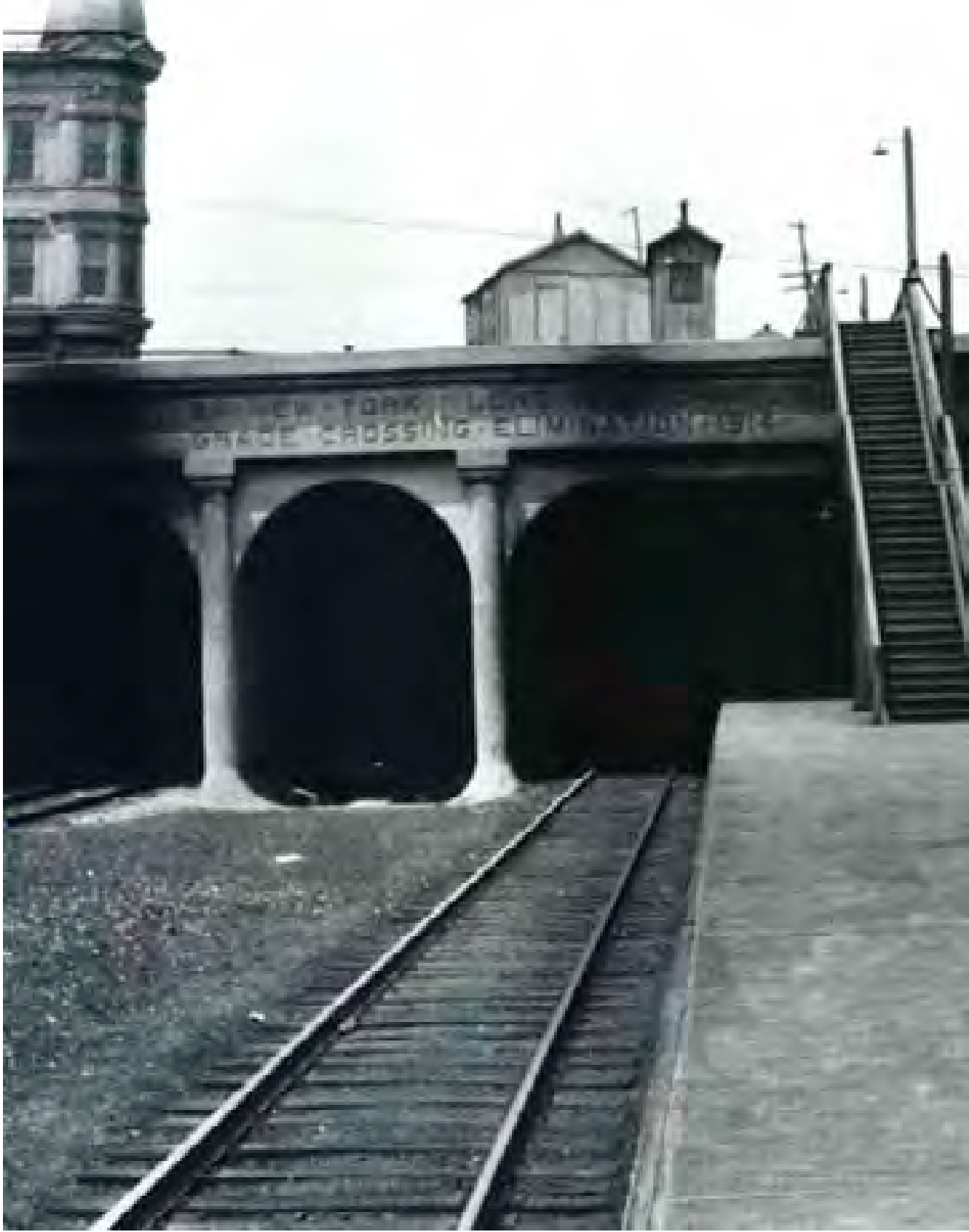
Kouwenhoven Station (now East New York Station), c. 1905.
