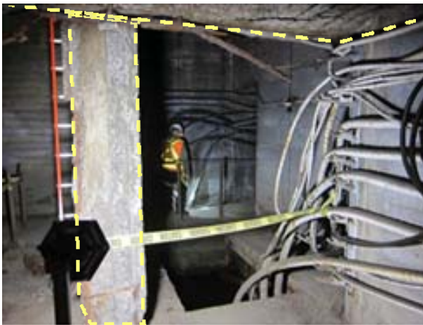
Column & beam repair
