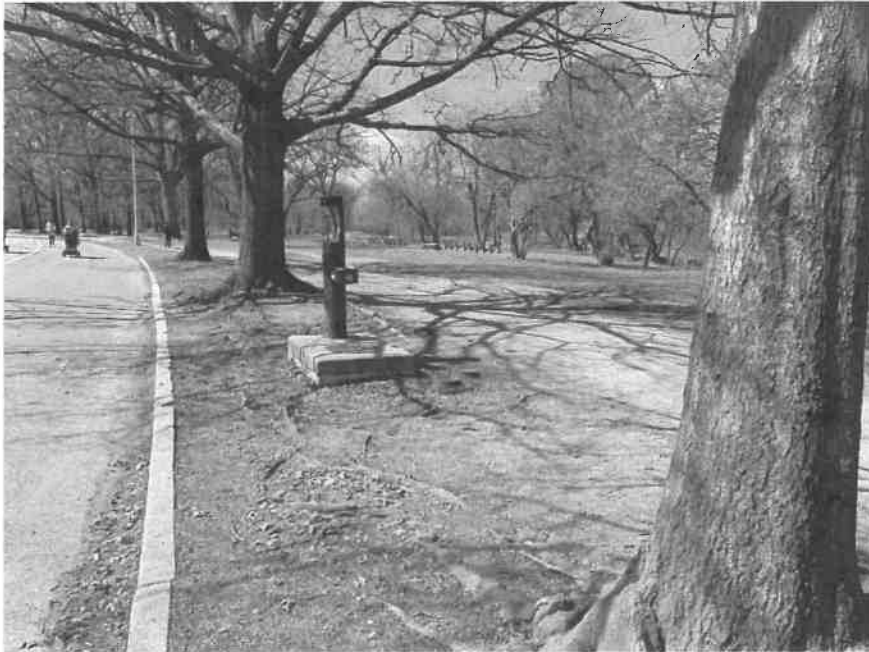
Heavy erosion around an inaccessible water bottle filler and drinking fountain
