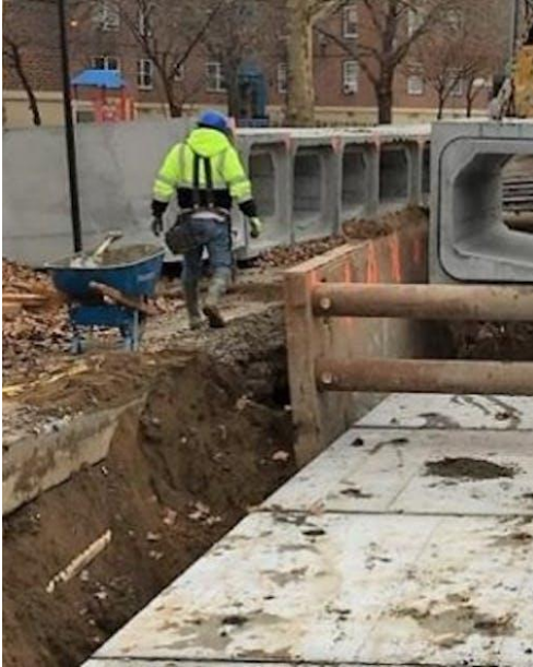
Expanding NYC's Sewer Drainage System
