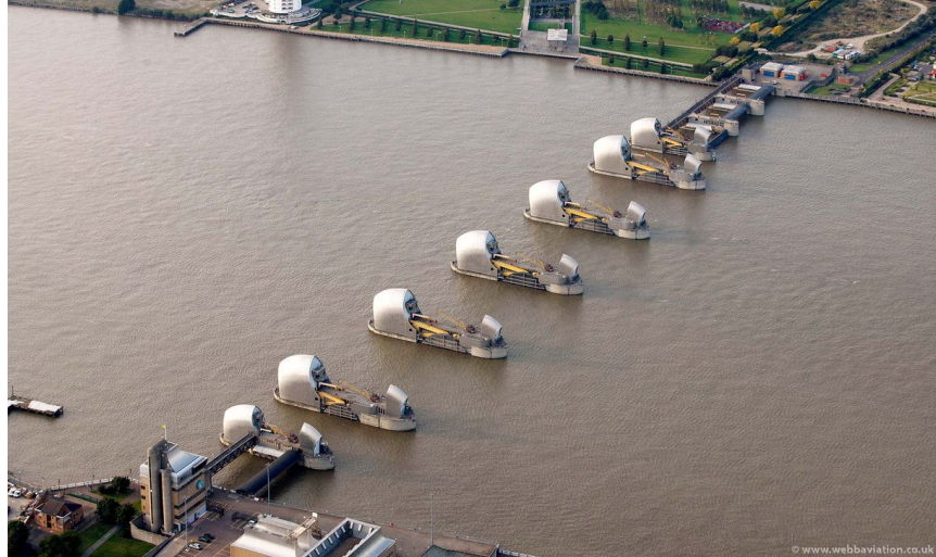
Other cities have or are currently building offshore moveable sea gate systems. River Thames, London, UK.
