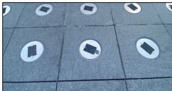
Example of flush element in pavement at spray area from Domino Park, Brooklyn
