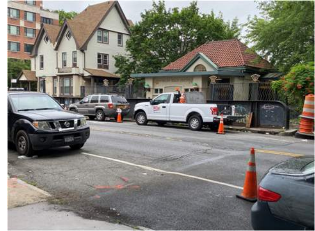
Subway Station Headhouse from Street
