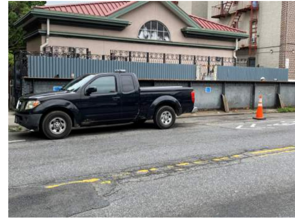
Existing Beam Along North Sidewalk
