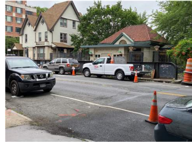
Subway Station Headhouse from Street
