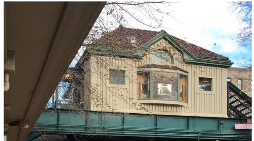
Subway Station Headhouse from Platform
