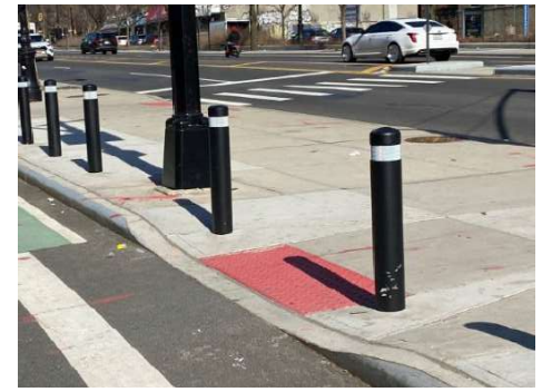
NYC DOT Pipe Bollard Dimension: 37 5/8" Ht., 5 9/16" diameter Color: Black
