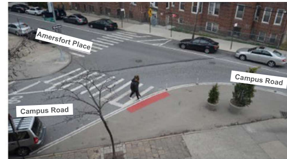
After 2016 SIP implementation, Campus Road and Amersfort Place, aerial view
