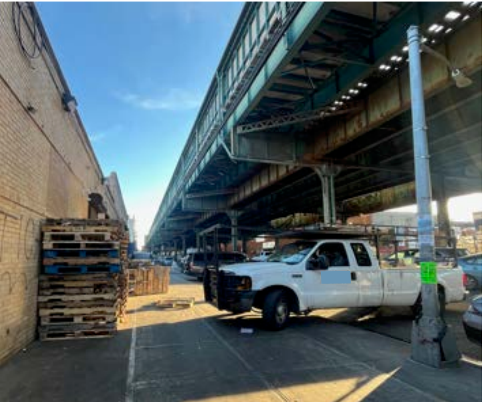
Challenging sidewalk conditions
